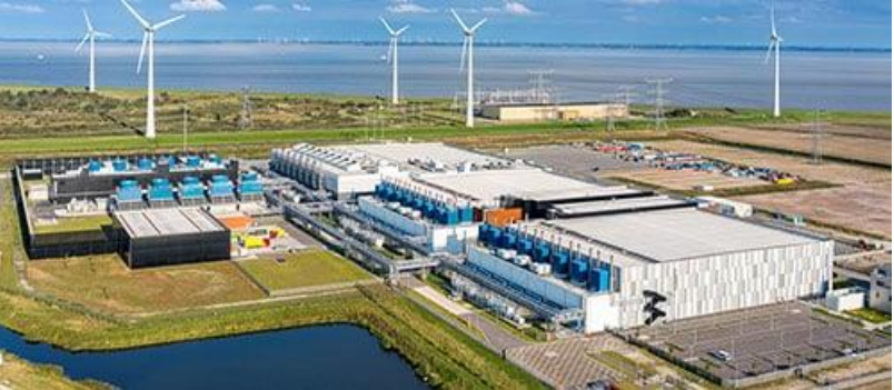
[Google Data Center, Eemshaven, Netherlands]
